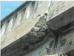
Concrete Deterioration with Exposed Rebar on the South Edge of the Deck over Bent 2
