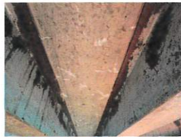
Typical Map Cracking with Efflorescence on Underside of Deck
