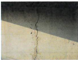
Typical Wide Vertical Crack on Backwalls
