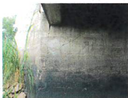
Cracking on the South End of the West Backwall
