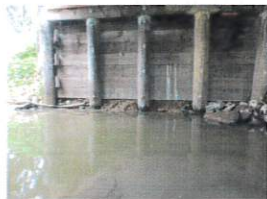
Undermining at the North End of the East Backwall
