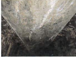
Typical Efflorescence and Stalactites on the underside of the Deck
