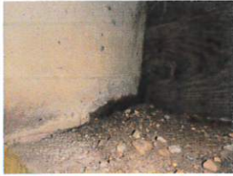
Spall on the North Leg of Unit 7 over Abutment 1
