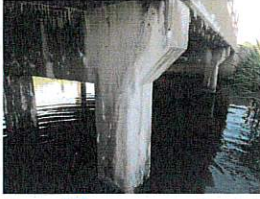
Heavy Efflorescence on the East End of Bent 2 (Typical to the West End of Bent 2)
