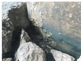
Concrete Deterioration at the North End of the East Backwall
