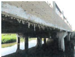
Heavy Efflorescence and Stalactites at the East end of Span 1 (Typical to the West End)
