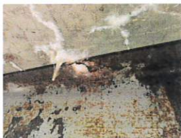
Typical Minor Section Loss Top Flange of Girders
