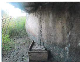
Cracking and Deterioration on North End of East Backwall
