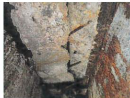
Concrete Deterioration in North Exterior Bay
