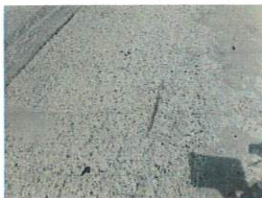
Exposed Rebar in Southeast Corner and Typical Scaling of Deck
