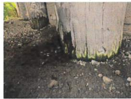
Typical Deterioration of Piles at the Ground line
