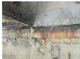
Typical Section Loss on the Bottom Flange of Girders 2-9 at Abutment 1
