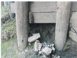
Undermining at the East End of the South Backwall
