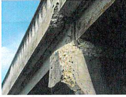
Concrete Deterioration at the South End of Bent Cap 2
