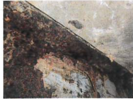
Typical Section Loss on Top Flanges of Girders
