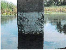
Poor Consolidation of Column 1 Bent 4
