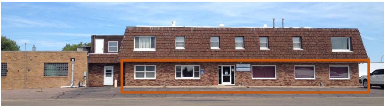
Figure 2: South entrance view.
