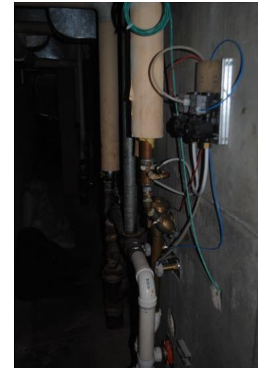
Close-up of the plumbing; uses precast form
